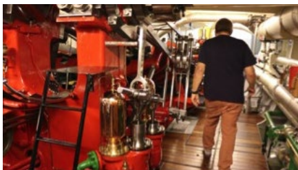
Figure 1: Salle des machines
